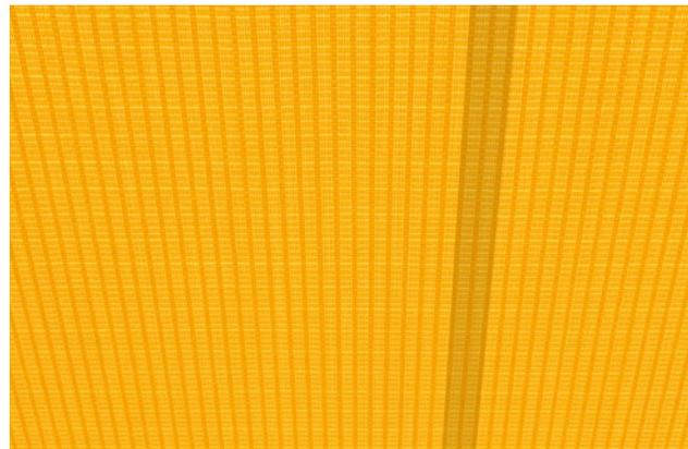
**Bonded awning covers** Panel joints bonded together ultrasonically ensure a consistent, unobtrusive appearance. Its excellent resistance to water, light and fluctuations in temperature ensures that the life expectancy of the cover is extended substantially.
